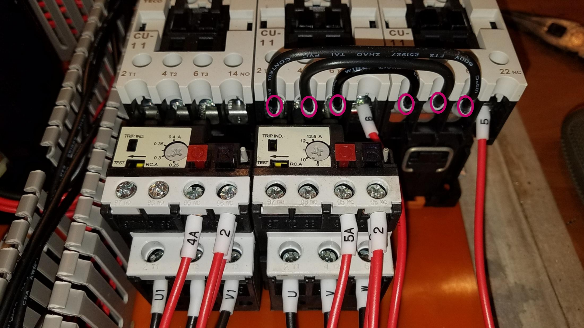
Remove the black jumper wires circled in purple between the forward and reverse contactors.
